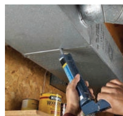
HVAC duct system
