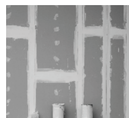
Construction joints
